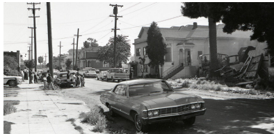
Children watch as a house is bulldozed in West Oakland, June 12, 1968.
